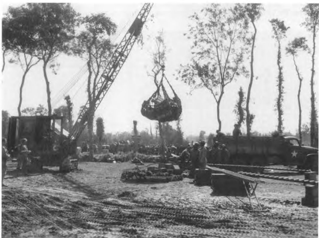
Using roller conveyor and other equipment to collect supplies stored behind the hedgerows, Normandy, 1944.
